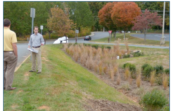
RRBC October 22 field trip: Dan Frisbee, Stormwater Coordinator for the City of Charlottesville, shows Commissioners the bio-swale at Charlottesville High School
